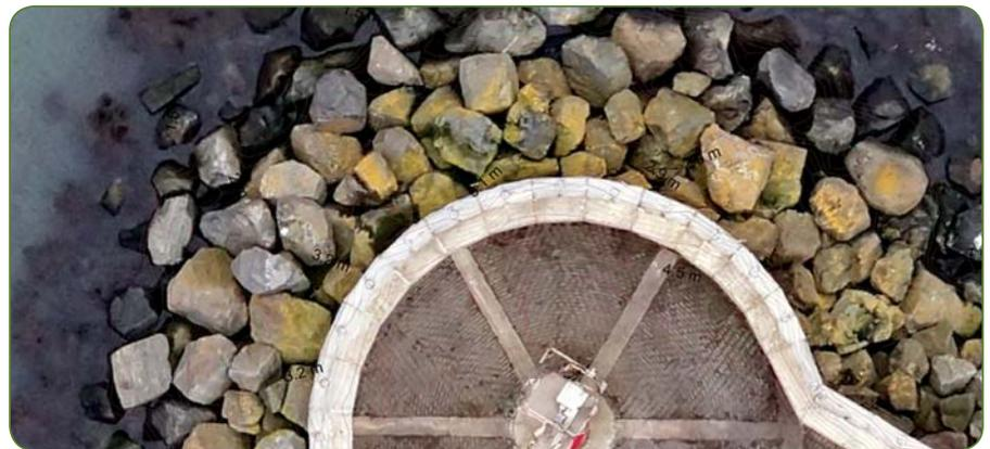
Fig. 4: Detail of revetment can be seen below at the pier head in our final output in AutoCAD.
